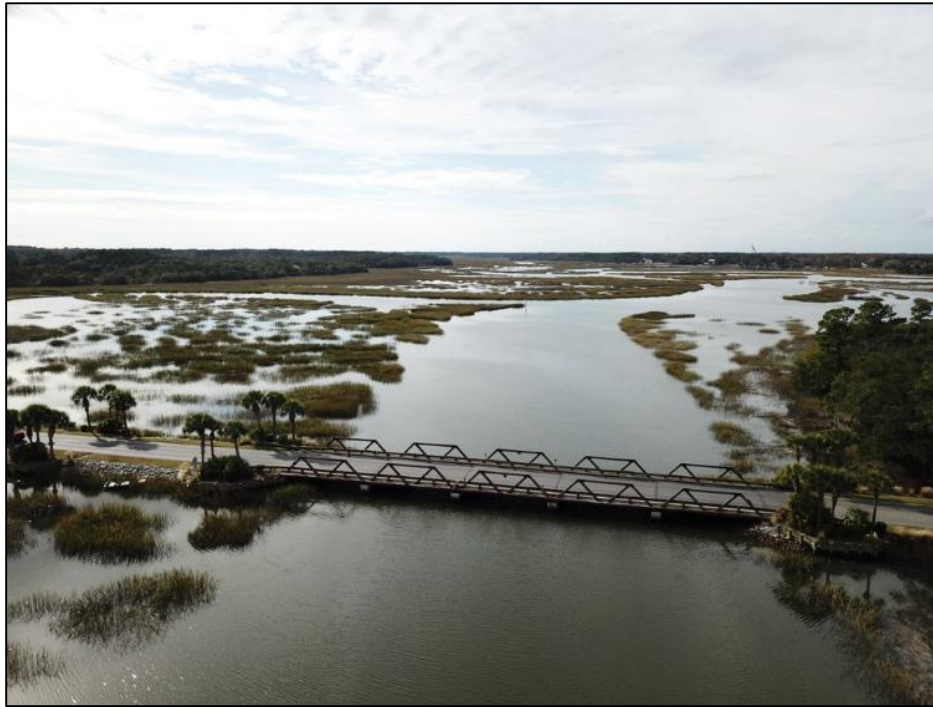
Figure 1-2: Existing Bridge Looking East
