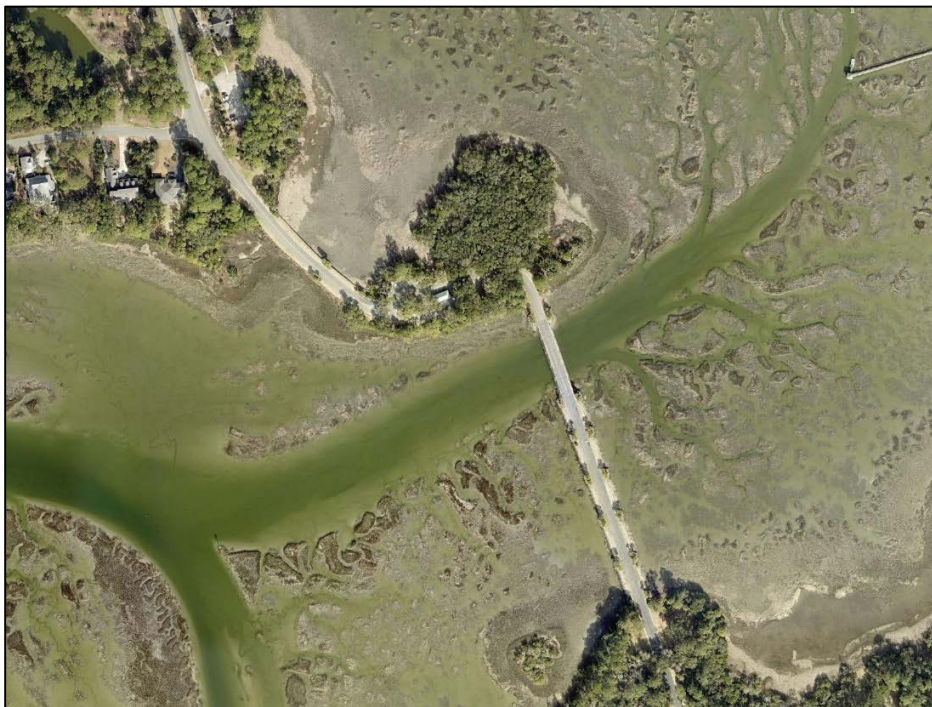
Figure 1-1: Aerial View of Existing Crossing
