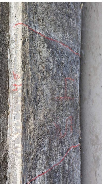
DEFECT 20: 1-9" Long, 1 Full Width Transverse Hairline Crack w/Efflo, 12"x3" Delamination at East Face of Patch
