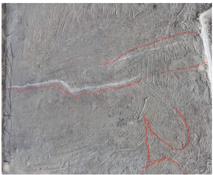
DEFECT 20: 1-9" Long, 1 Full Width Transverse Hairline Crack w/Efflo, 12"x3" Delamination at East Face of Patch
