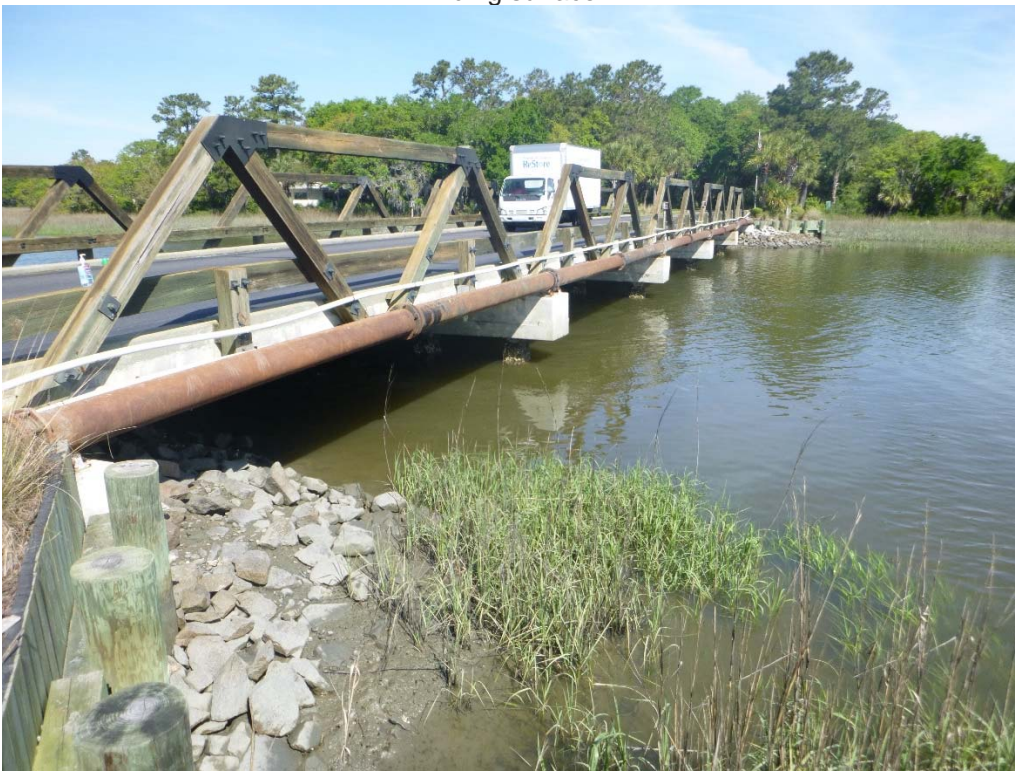
Bridge profile/Cap repairs
