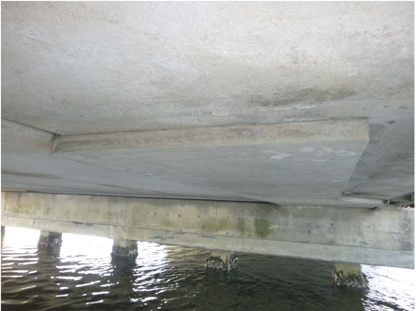
Special panel repair location
